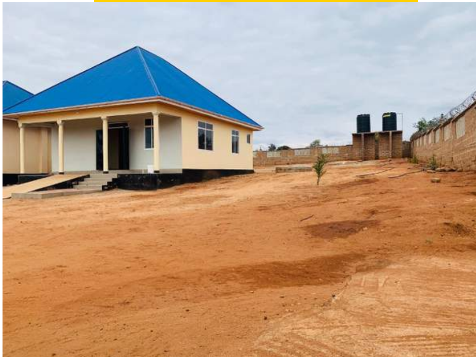
Front of the Office building
